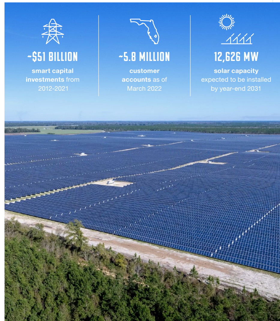
The Blue Springs Solar Energy Center is one of the newer solar installations in the FPL fleet. The facility, located in Northwest Florida's Jackson County, was commissioned in 2022.
