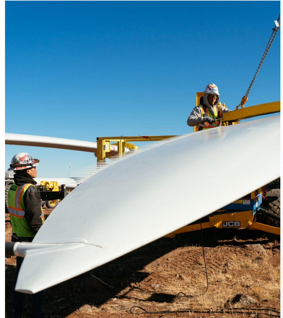
Crew members team up to install new wind generating equipment during construction of the Borderlands Wind Energy Center in Quemado, N.M.
