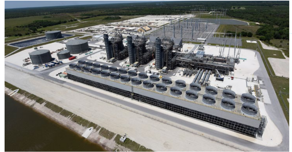
Environmental water conservation measures are underway at the Okeechobee Clean Energy Center in Florida to deepen a groundwater well which will allow the company to reduce its potable ground water use at this site.
