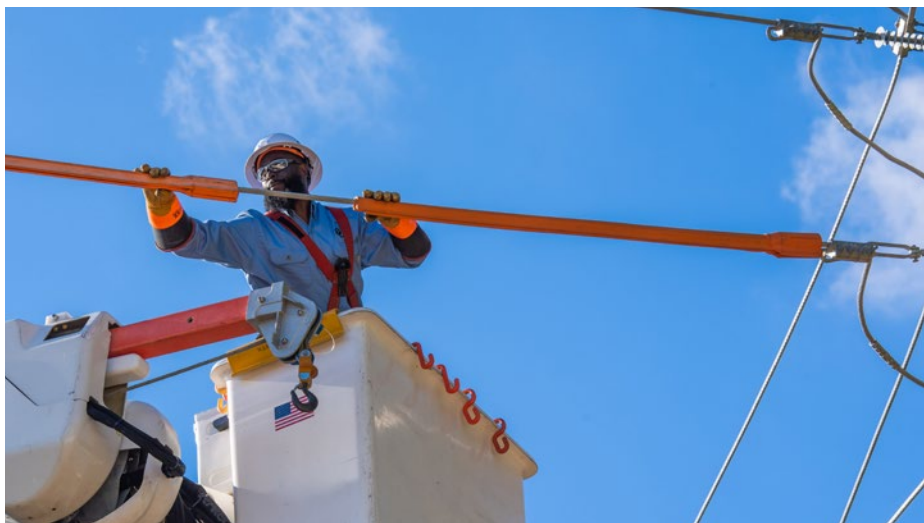
Arlo Smith works on a storm hardening project in Northwest Florida.
