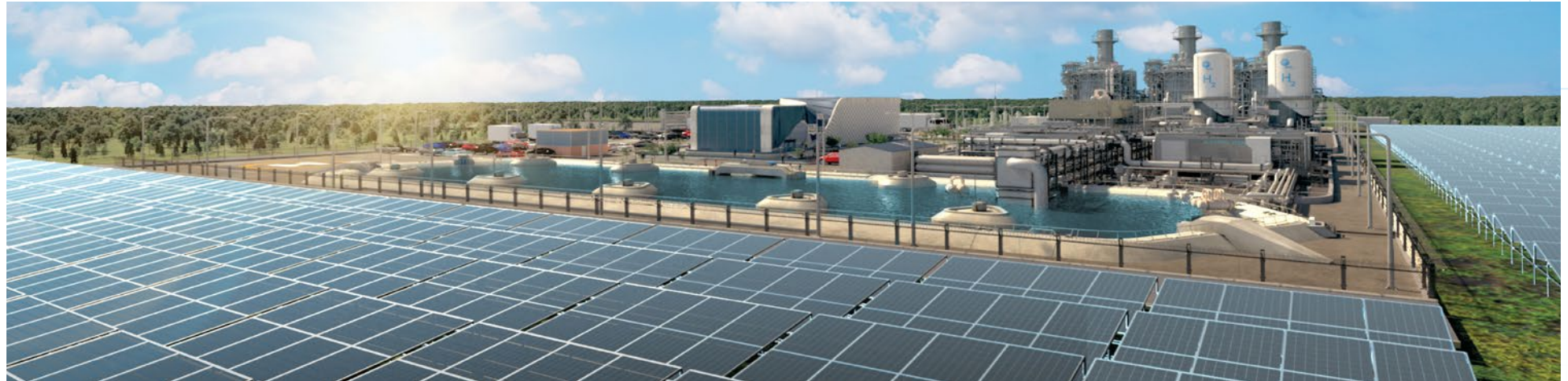
An artist's rendering of the Okeechobee Clean Energy Center in Florida includes the Cavendish NextGen Hydrogen Hub.
